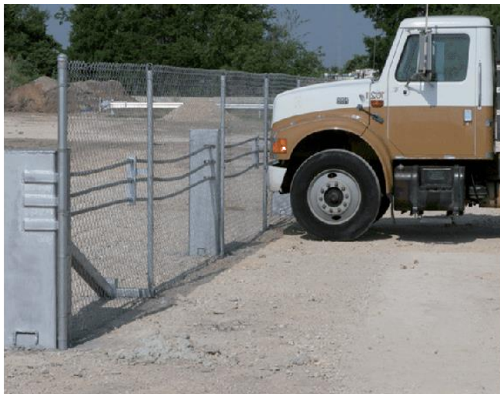
Figure 5: Cable reinforced fence
